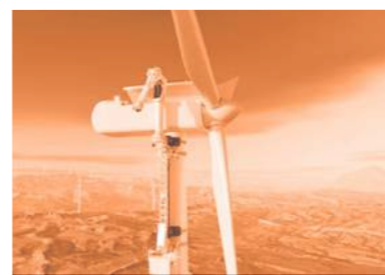
Windmill Service crane
